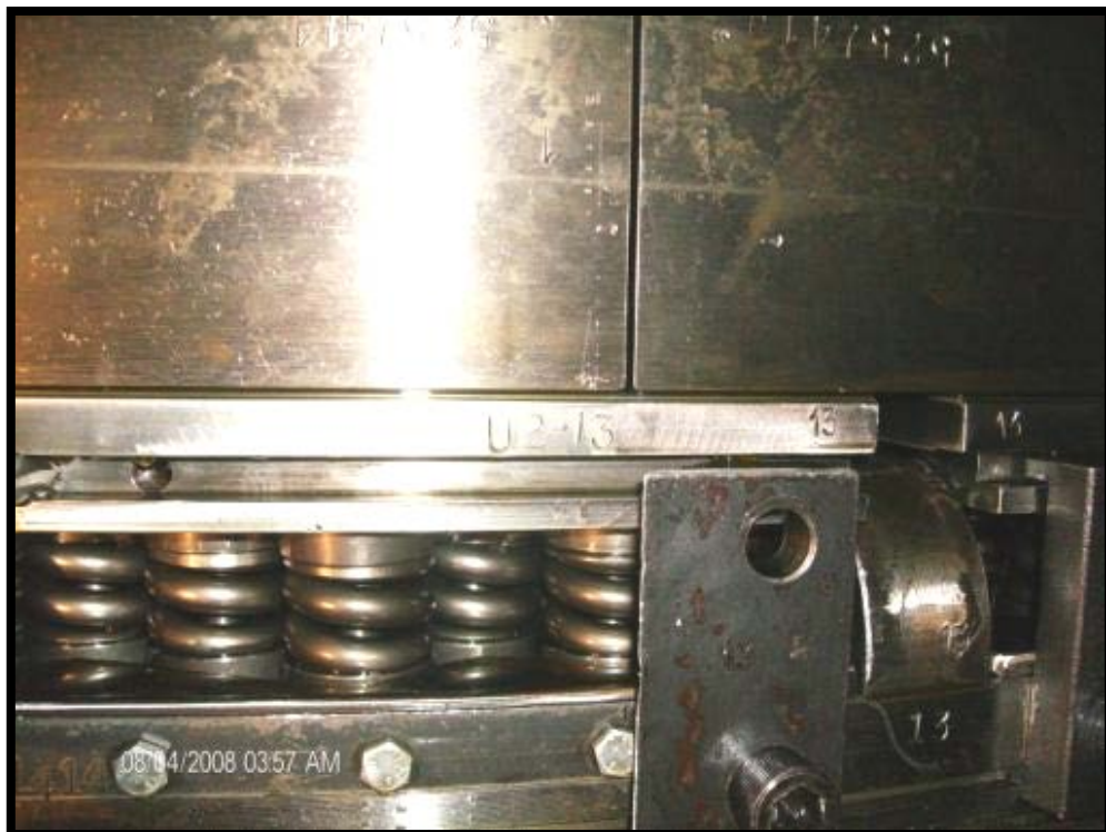
Photo 2 Old Runner Plate With Gap Between Segments
