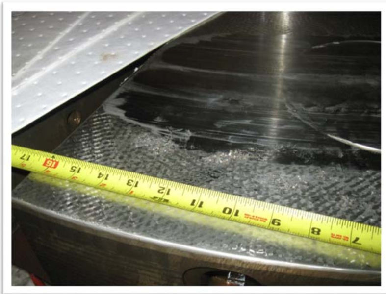
Photo 5: Wiped thrust bearing
