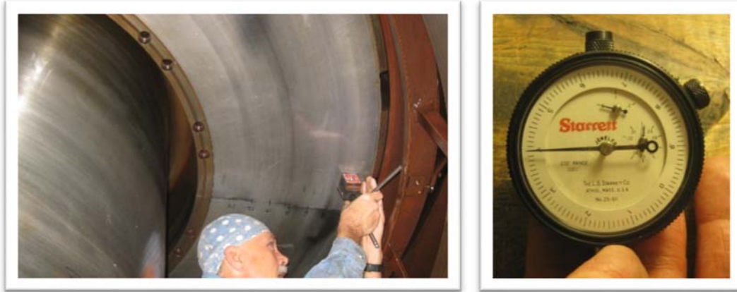
Photo 6 & 7: Sweeping the thrust runner split with a 0.0001 inch dial indicator
