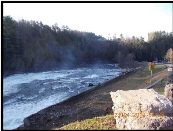
Looking down penstock towards powerhouse
