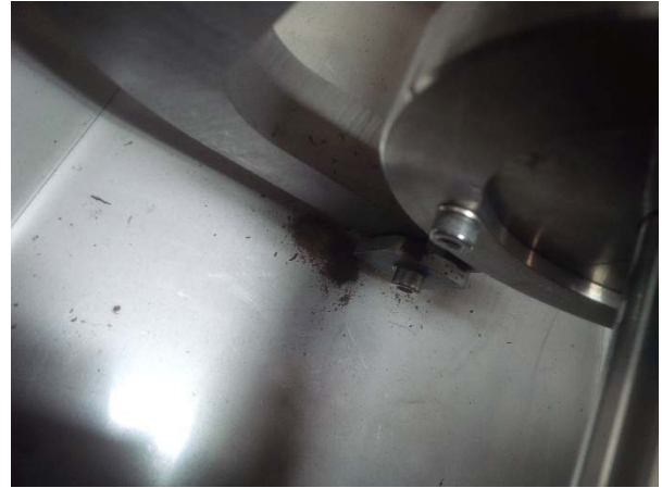
Photo 25: Worn L/V material under ring #1
