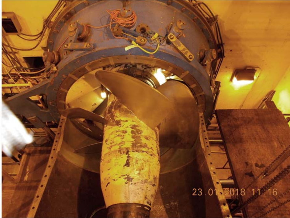
Photo 1: Turbine with discharge ring removed for access to seal area
