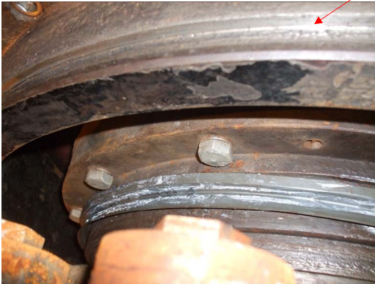
Photos 2a & 2b: Inner seal ring cleaned and installed
